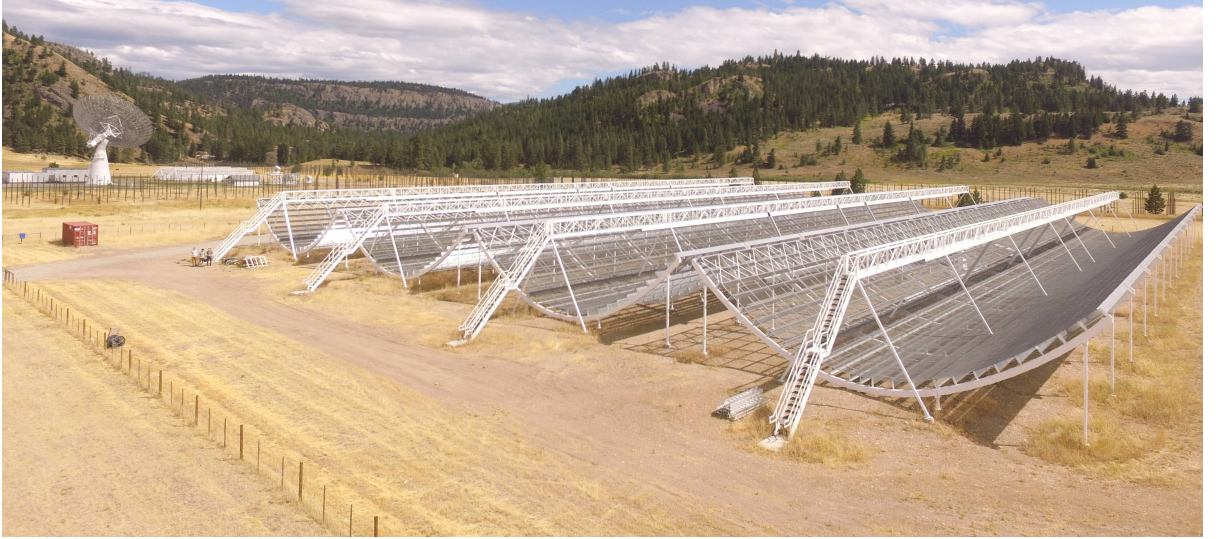
Figure 1.3: Canadian Hydrogen Intensity Mapping Experiment in Penticton, British Columbia, Canada, in the South-East direction. The four cylindrical reflectors lay along the North-South direction and each have 256 dual polarization feeds at their focal line. The 26 m Galt telescope is visible on the left. Drone image courtesy of CHIME Collaboration.
